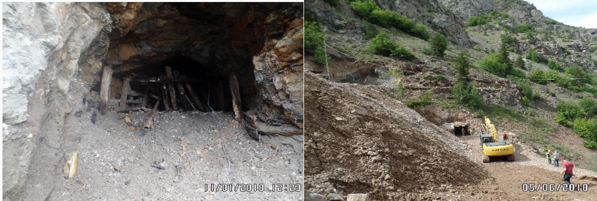
Figure 7. Yavuz TÜRKEK, The views from underground gallery works
